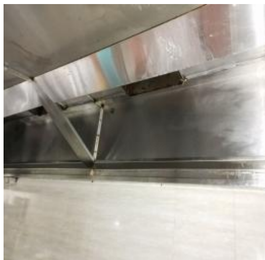
烧腊房烟罩清洗后
