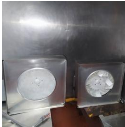
烧腊厨房风轮清洗后
