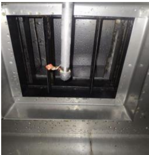
烧腊房烟罩清洗后 1
