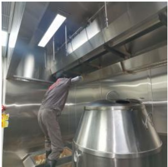
烧腊房烟罩施工
