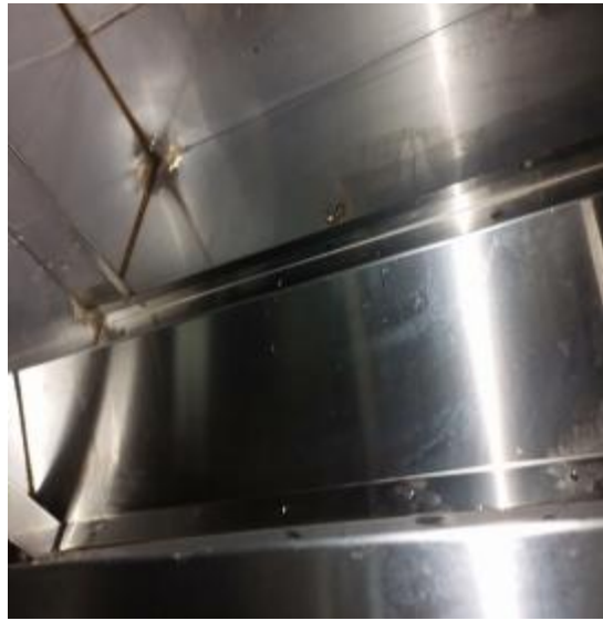
烧腊房烟罩清洗后
