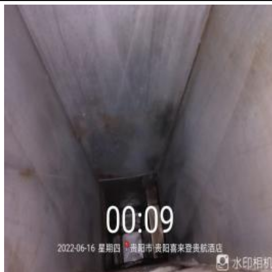
烧腊管道清洗后
