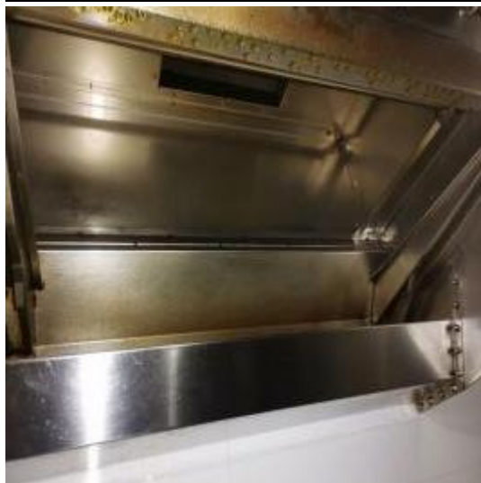
烧腊房烟罩清洗前
