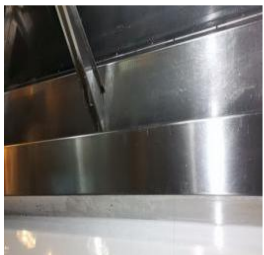
烧腊房油槽清洗后
