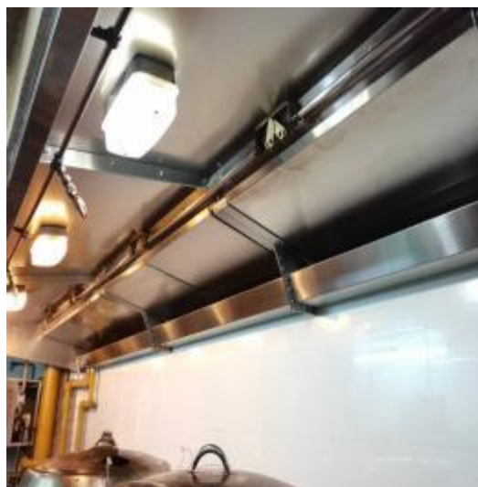
烧腊房烟罩清洗后
