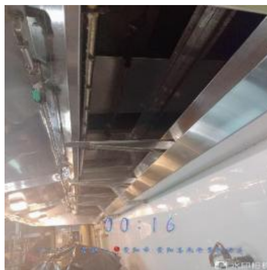
烧腊房烟罩清洗后
