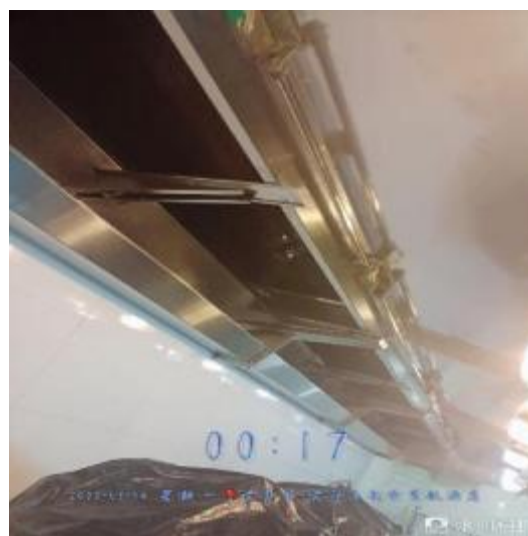
烧腊房烟罩清洗后
