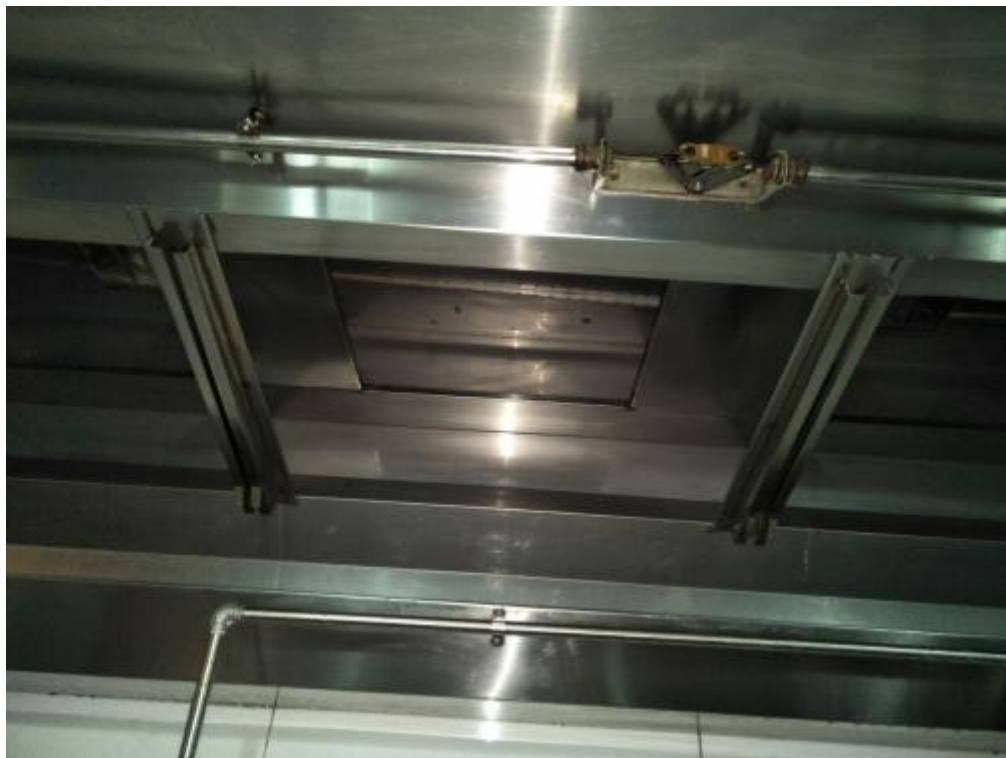
烧腊房烟罩施工后
