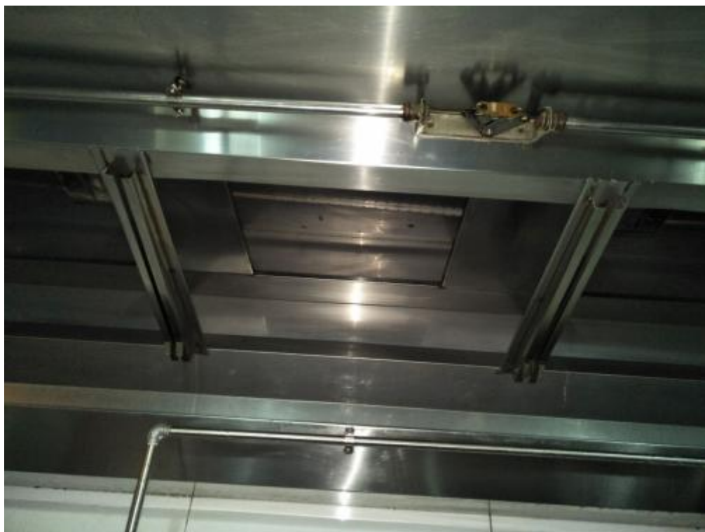
烧腊房烟罩施工后
