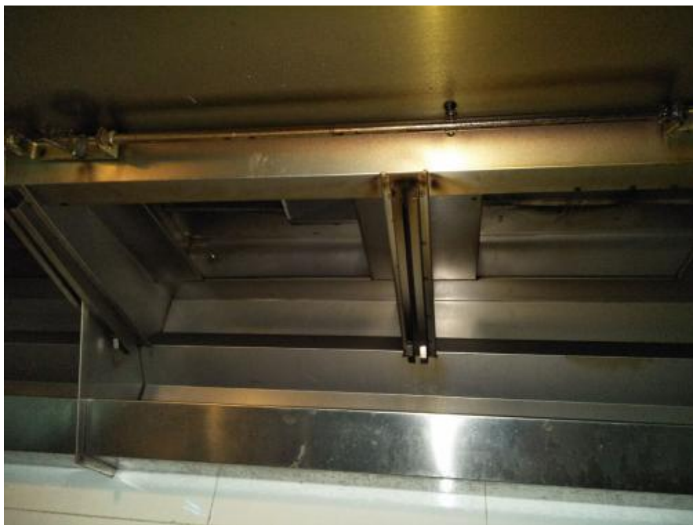
烧腊房烟罩施工前
