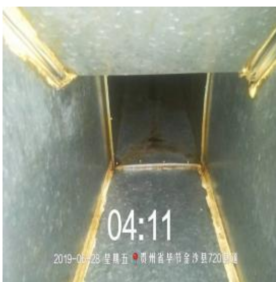
翘脚牛肉主管道清洗后 1
