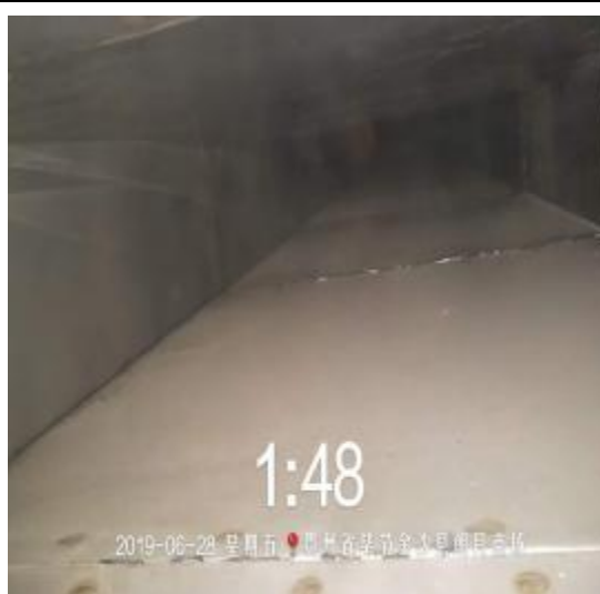
翘脚牛肉主管道清洗后 2
